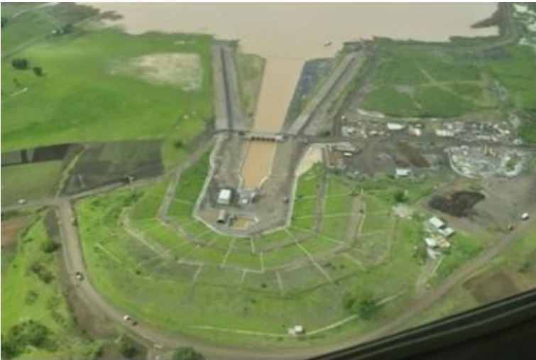
APPROACH CHANNEL TO THE INTAKE TUNNEL
